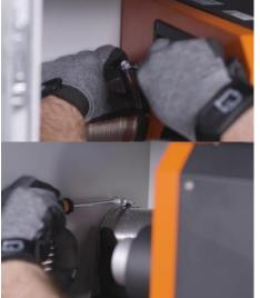
Fasten the corrugated aluminum pipe ( $\emptyset$  100 mm) with the pipe clamps ( $\emptyset$  100 mm) to the black inlet air socket of the Ecoport and the passage to the outside
