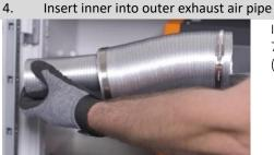
Insert the narrower corrugated aluminum tube ( $\emptyset$  70 mm) into the wider corrugated aluminum tube ( $\emptyset$  100 mm).
