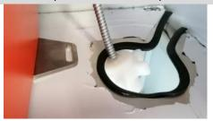
Guide the tank supply line of the Ecoport through the prepared breakthrough (approx.  $\emptyset$  100 mm).
