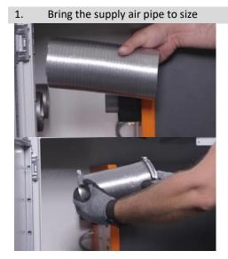
Bring the corrugated aluminum pipe (Ø 100 mm) to the appropriate length between the black inlet air socket of the Ecoport and the passage to the outside by pulling it out or cutting it to size
