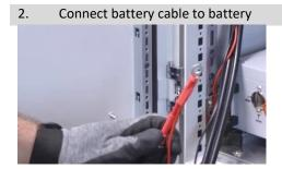
The red contact of the battery cable must be connected to the positive pole (+) of the battery.
