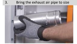
By extending or cutting to size, bring the two corrugated aluminum pipes ( $\emptyset$  100 mm &  $\emptyset$  70 mm) to the appropriate length between the black exhaust air socket of the Ecoport and the passage to the outside.
