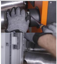
Fix the outer corrugated aluminum pipe ( $\emptyset$  100 mm) on both sides with one pipe clamp each.
