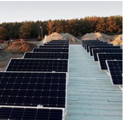
Installation in a gravel pit in Southern Germany. In the energy system, a combination of fuel cell, PV, and battery reliably supplies energy for an office container – offering an environmentally friendly off-grid power supply.
